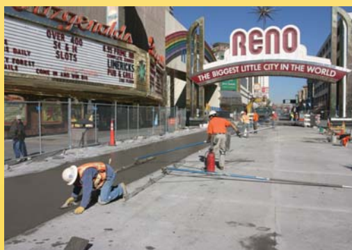
Reno chose decorative concrete pavement for a much-needed facelift for its downtown shopping district. (Photo: Granite Construction)
