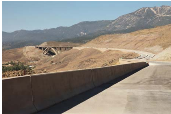
New concrete pavement and Galena Creek Bridge.
