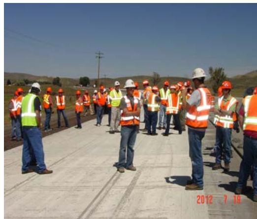
Concrete overlay open house in Wyoming.
