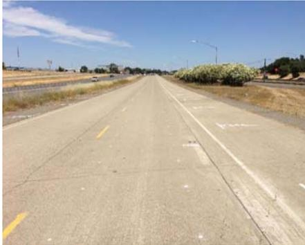
Caltrans has announced the opening of California's first certification and calibration site for inertial profiler devices and technicians. Caltrans is moving to update its pavement smoothness specifications to accommodate new measurement technology. The site is located in Sacramento at the Watt Avenue Light Rail station. The concrete pavement section is jointed plain concrete.
