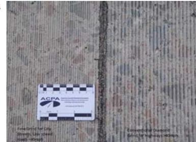
SWCPA has proposed this texture as a way to smooth out old, faulted pavements in the Los Angeles Hancock Park neighborhood area. The new texture is achieved with diamond grinding equipment that will level the surface of existing concrete pavements while providing a surface with fine grooves that yield a slip-resistant surface. The surface is designed for low speed roads and the smooth, fine-groove surface makes it ideal for bicycles and skateboards.
