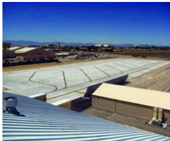
Completed ramp at Edwards Air Force Base, Calif.
